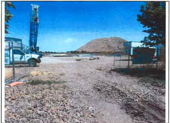
22. View north of equipment storage area in southwest portion of subject property (temporary lease by contractor at adjacent south construction site).
