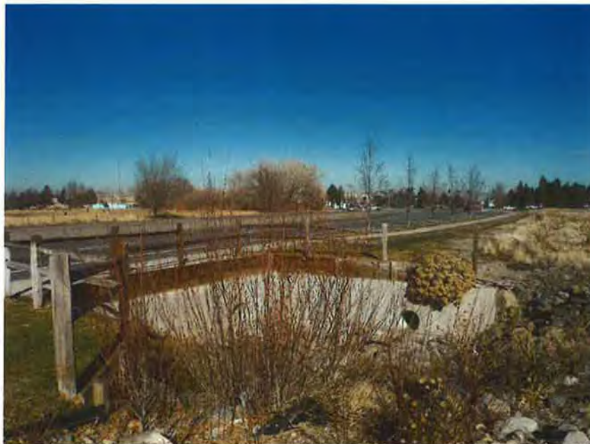
Photo 2 – Larger storm drain along Longley Lane
