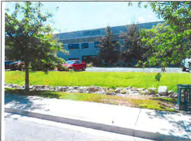
33. View of adjacent property to south (central portion) across Innovation Drive, warehouses/offices flex building.
