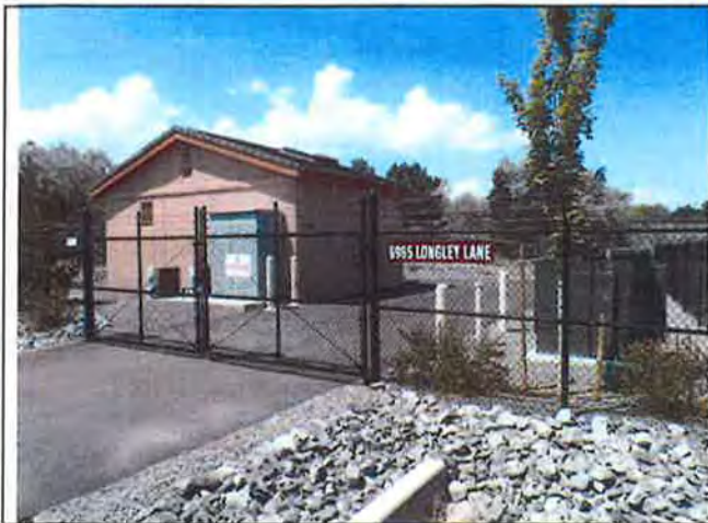
35. View of adjacent property to southwest across Longley Lane, utility station.
